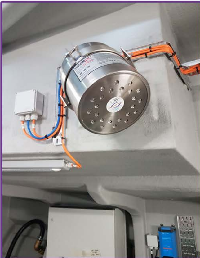
Explanation of the extinguishing device installation and its connection to the electrical current
